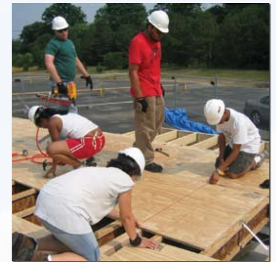
Sheer Wall & Sub Floor
