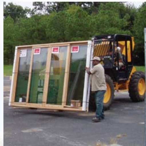
Doors and Windows
